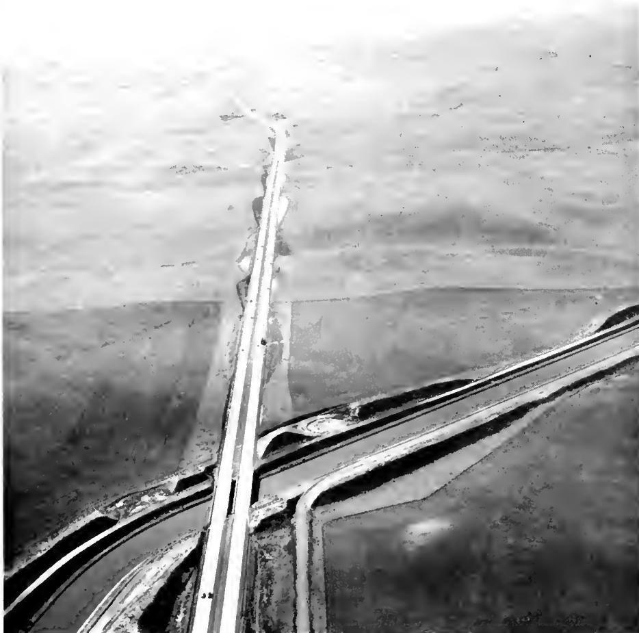
Expressway on US 50 at crossing of the Delta Mendota Canal near the Alameda-San Joaquin County line. New construction joins with the original four-lane divided facility through the Altamont Pass in the distance where the ramps of an interchange are discernible.
